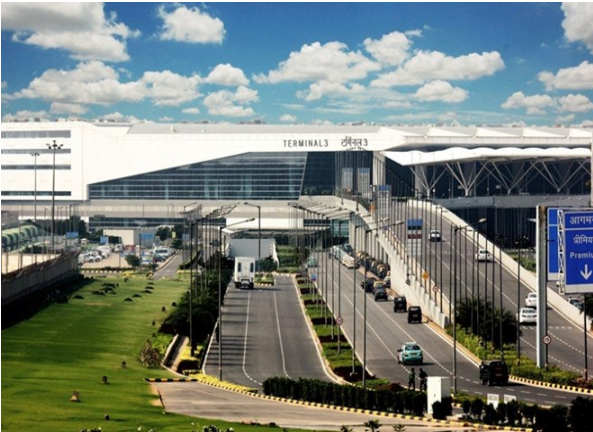
Figure 1. Terminal 3 of Indira Gandhi International Airport
