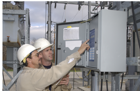
Figure 2. Routine inspection of substations
