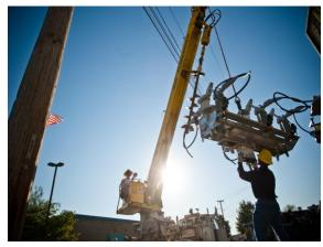
Figure 2: Installation of Smart Switches across EPB distribution network
